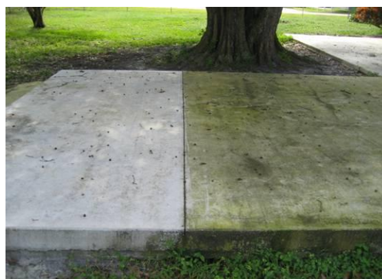
Figure 4: Images of existing concrete slabs: DCE-treated (left) and untreated (right). No cleaning was made to the surface prior to applying the DCE technology.
